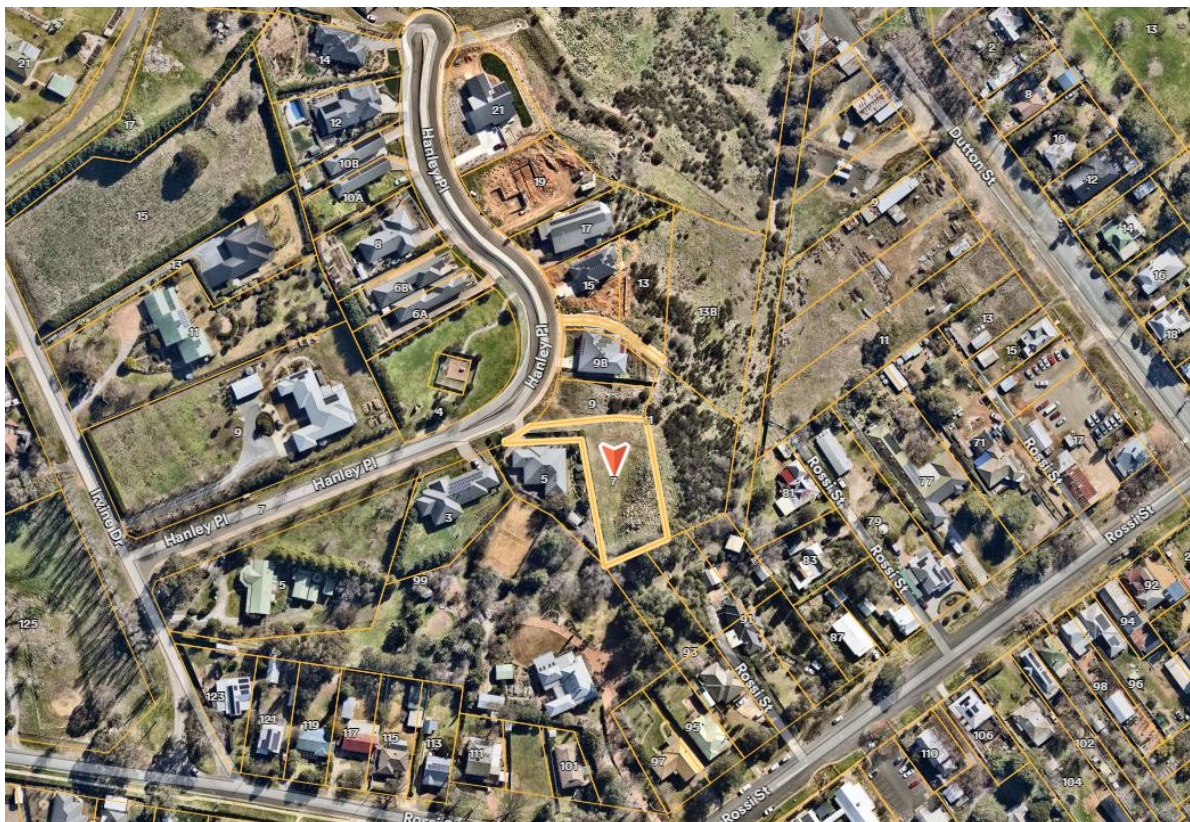
Figure 2 – Aerial view of subject site in its immediate context. Source: Nearmap.
