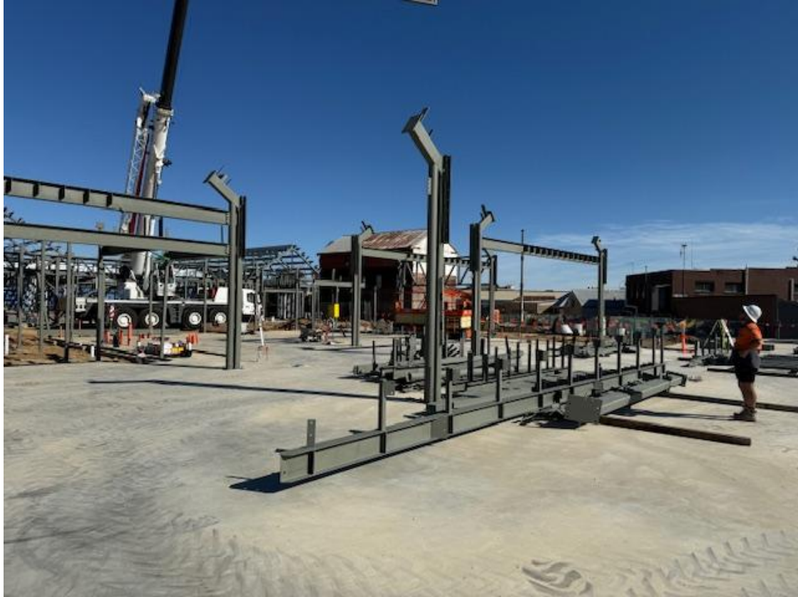
Figure 2 & 3 Admin Structural Steel installation
