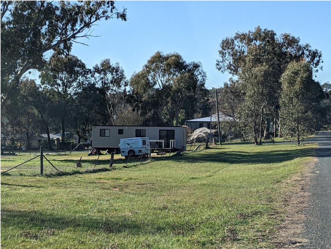
Figure 2 – Dwelling as viewed from Woolrych Street (Facing North)
