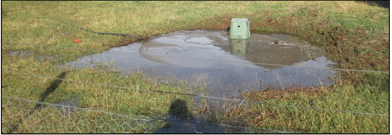
Figure 2: Inundated Septic System
