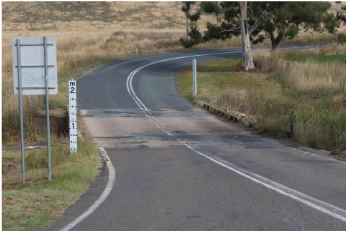
Causeway (Note: no side rails only concrete blocks (with a number missing) to prevent vehicles from going over the edge)
