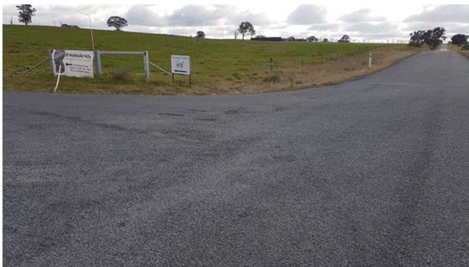
Figure 7 - Junction Southwell and Brooklands - pavement thinning and failure - looking Northwest
