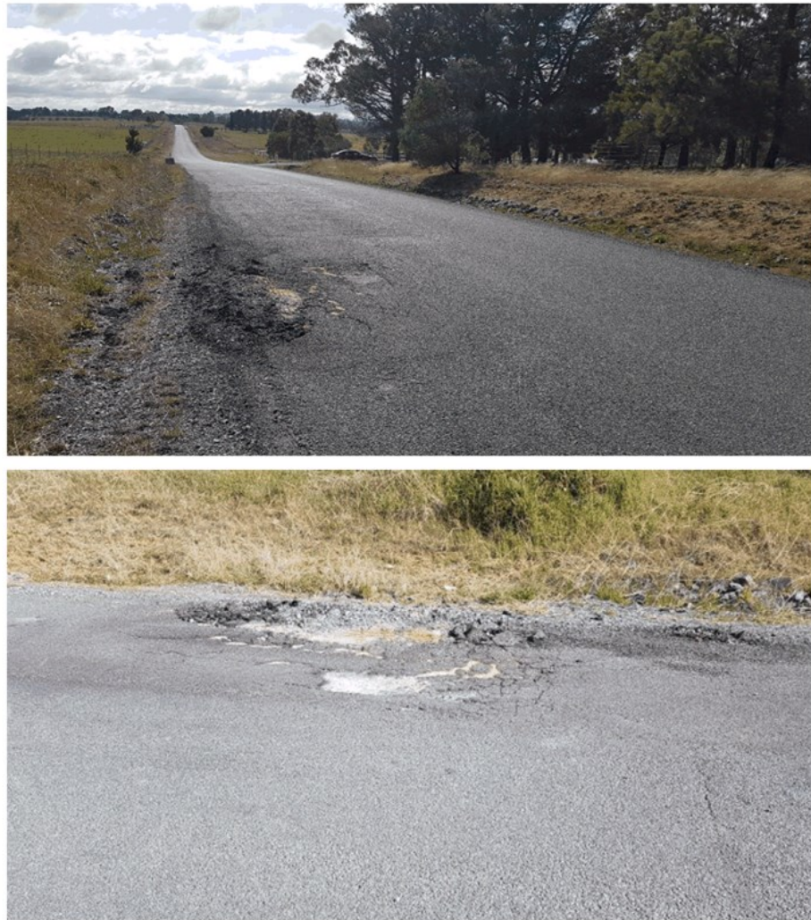
Figure 5 (a and b)- Pothole and pavement failure (long-term and reoccurring) in front of 93 Southwell Rd (note driveway in mid-ground to the right)
