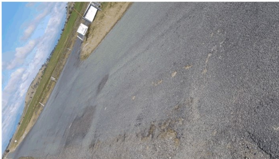
Figure 6 - Junction Southwell and Brooklands - pavement thinning and failure - looking Southwest
