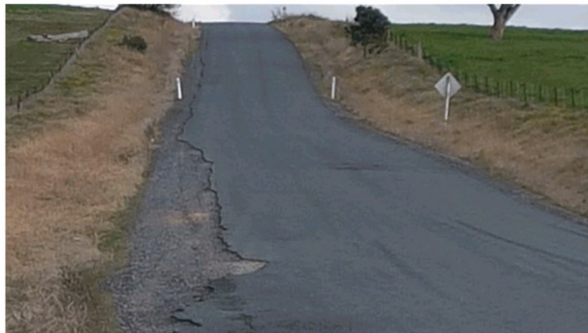
Figure 8 - Brooklands Road from Southwell looking West with shoulder failure
